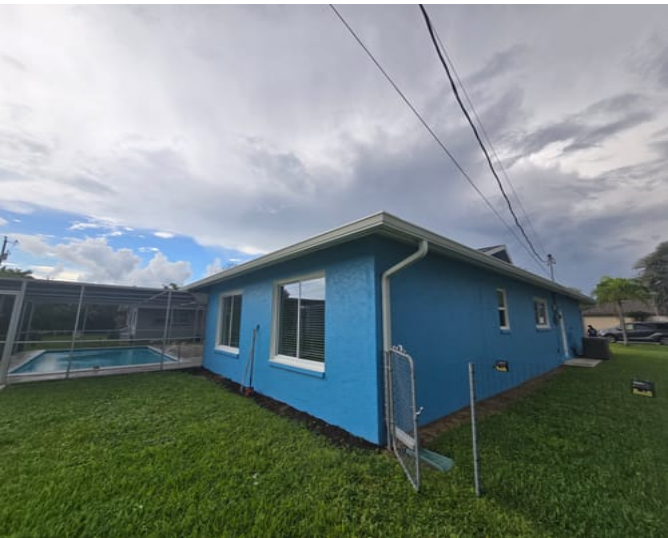
Photo 3 - Side of Home
