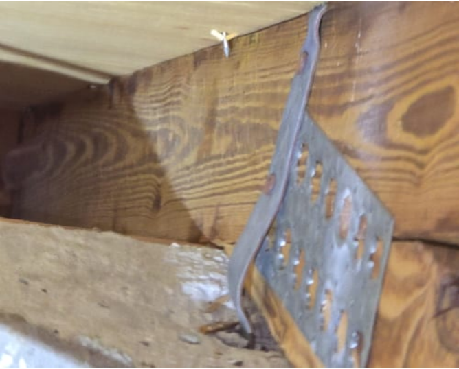
Photo 2 - Hurricane Clips/Straps
