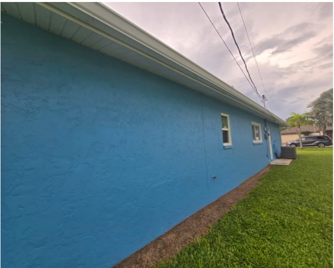
Photo 4 - Side of Home
