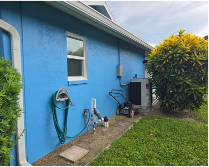
Photo 2 - Side of Home
