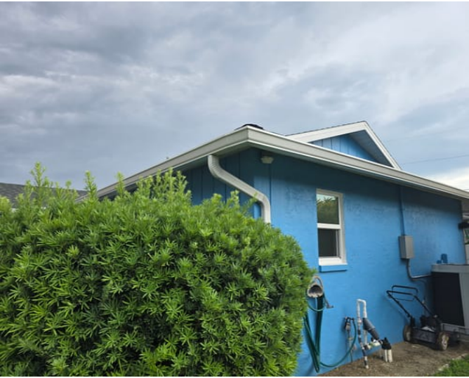
Photo 1 - Side of Home
