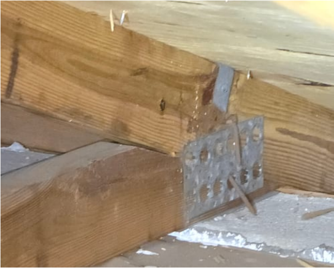
Photo 1 - Hurricane Clips/Straps
