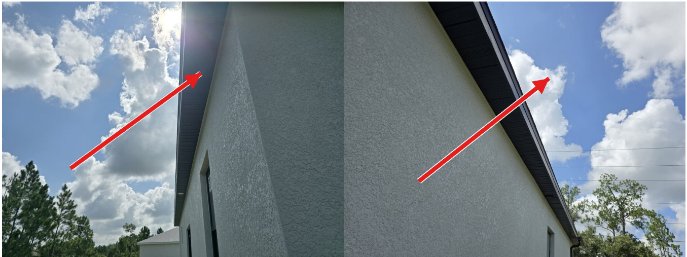
Fachada sin canal / Elevation without gutter
