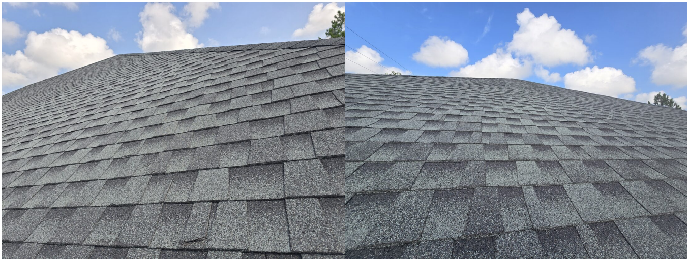
Cubierta general / General roof covering
