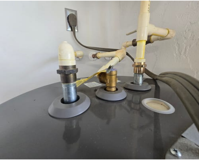
Photo 1 - Temperature Pressure Relief (TPR)
