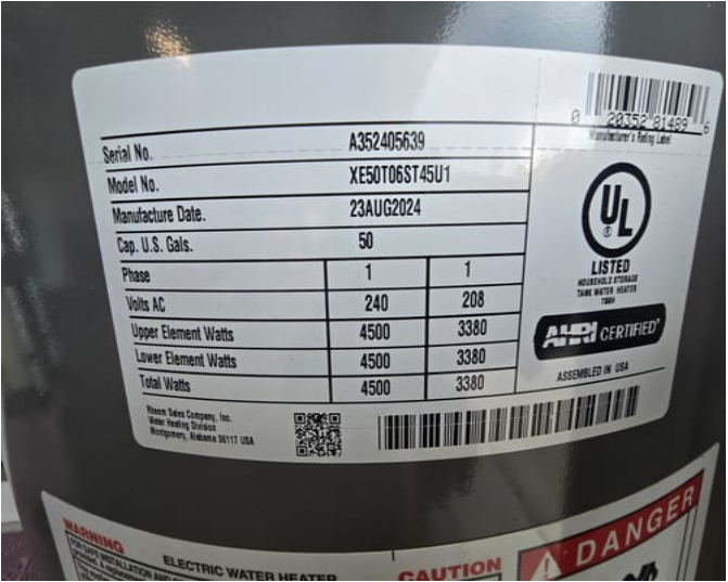
Photo 1 - Water Heater Label
